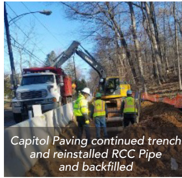
Capitol Paving continued trenching and reinstalling RCC Pipe for storm drainage
